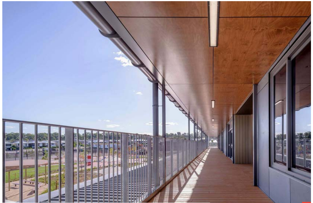
1/ Austral Ply supplied more than 200 sq m of Ariaply panels that were adhesive-fixed to metal framing.
