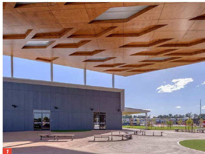
1/ Austral Ply supplied more than 200 sq m of Ariaply panels that were adhesive-fixed to metal framing.
