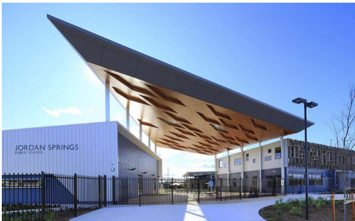
Plywood panels finished in a unique three-coast system at Jordan Springs provided durability and an attractive outward appearance for the school’s modular buildings. Photos: Modscape and Richard Crookes Constructions
