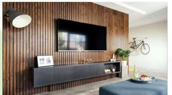
Installing the panels with a 10mm "express joint" is an attractive method that presents the panels best. Paint the gaps black before installing the panels to emphasize the joint.
