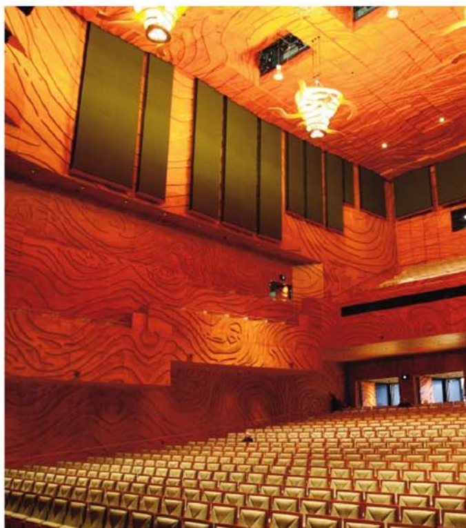
Hoop pine laminated panels a key inside feature of the $75 million Melbourne Recital Centre.
